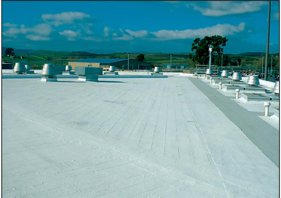
■ This white, highly reflective acrylic roof coating is applied at a heavy coverage rate directly over a three-ply BUR system.
