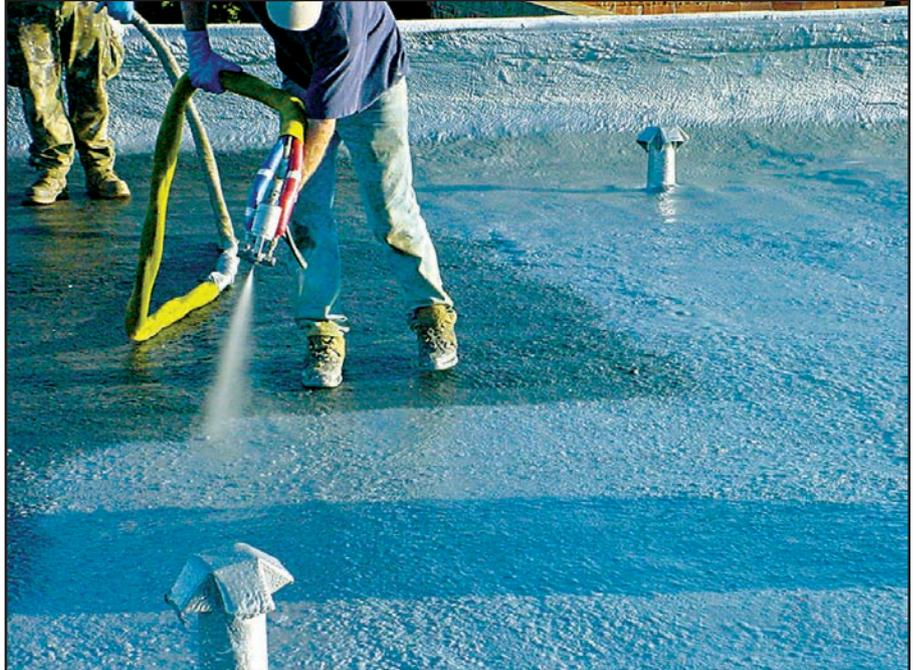
■ In this photo, a roof contractor is using plural component spray equipment to recoat an existing SPF system with a two-component polyurea coating over a urethane primer. This polyurea coating cures within 30 seconds of application.
