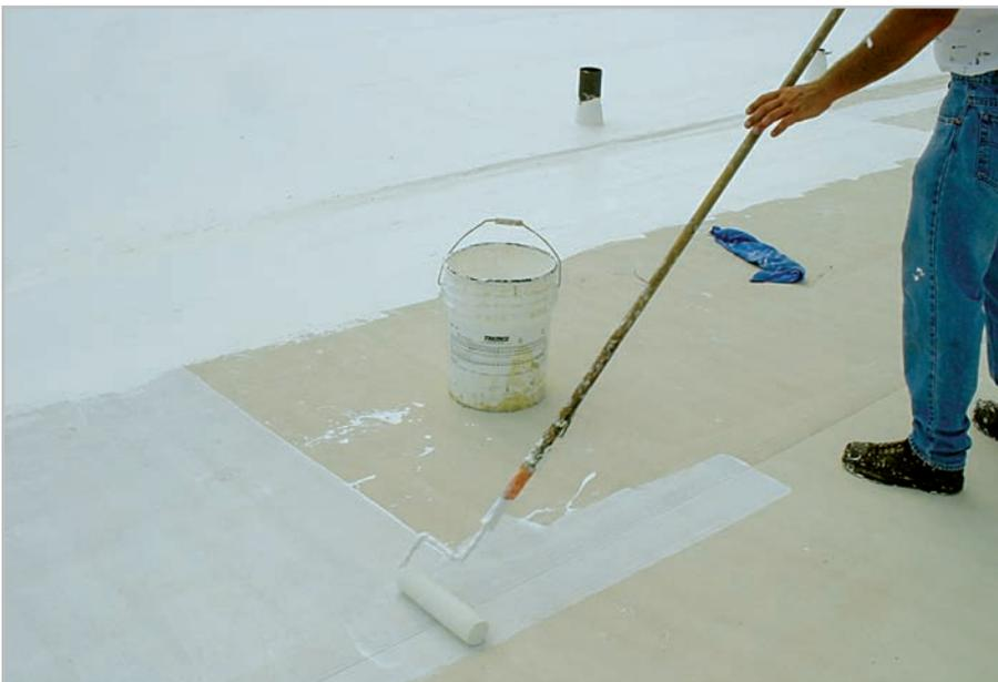
■ Here a roof contractor is roller applying a water-based primer and acrylic coating as a restoration coating over an existing reinforced CSPE single-ply roof system. This coating system was specified for use over this refrigerated food storage facility due to the low odor features of the coating and excellent bond strength of this primer.
