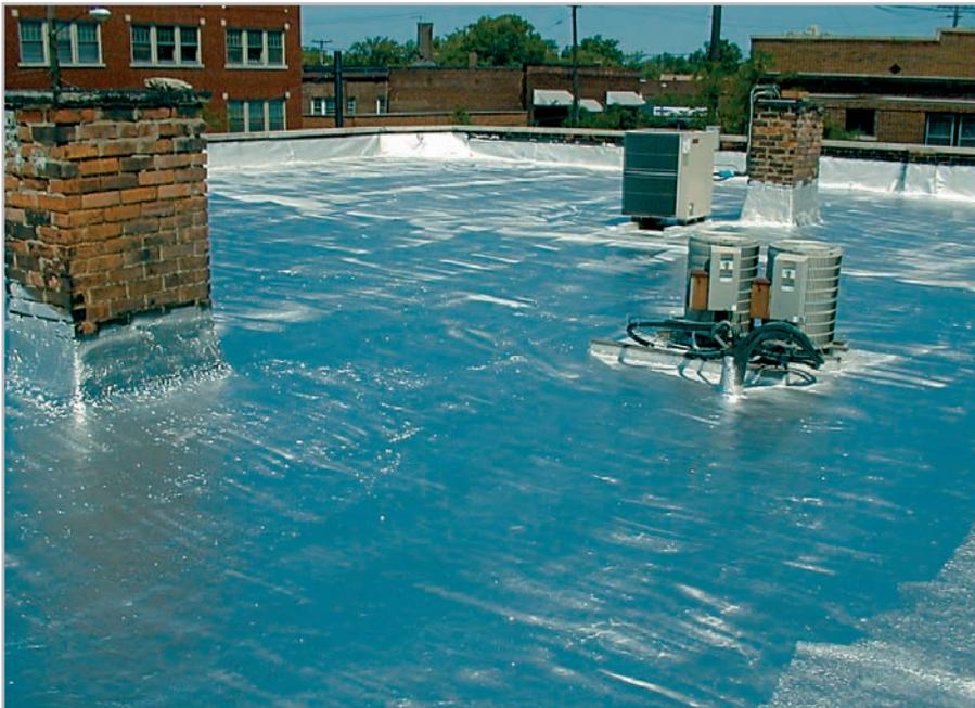
■ This solvent-based aluminum coating was applied over an asphalt emulsion surfacing over a smooth asphalt cold process BUR system. This roof manufacturer's surfacing system is UL fire rated over a variety of roof systems.
